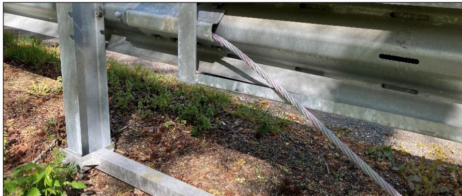
Figure 13: Guardrail in the curves near Vertical Ridge Road
