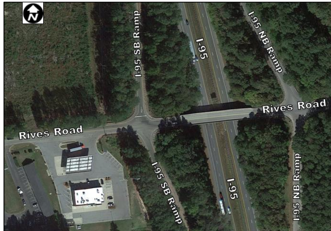
FIGURE 1.12. RIVES ROAD AND I-95 SOUTHBOUND RAMP
