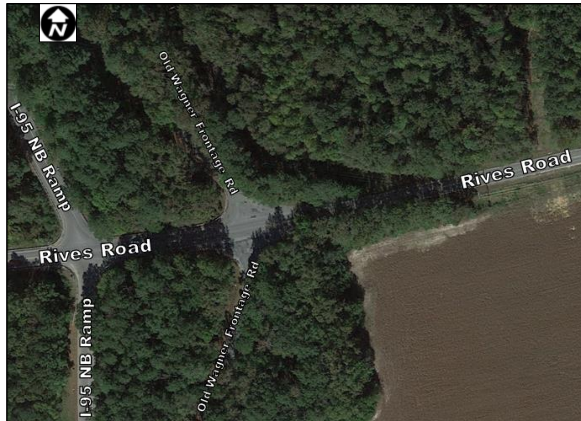
FIGURE 1.14. RIVES RD AND OLD WAGNER FRONTAGE ROAD
