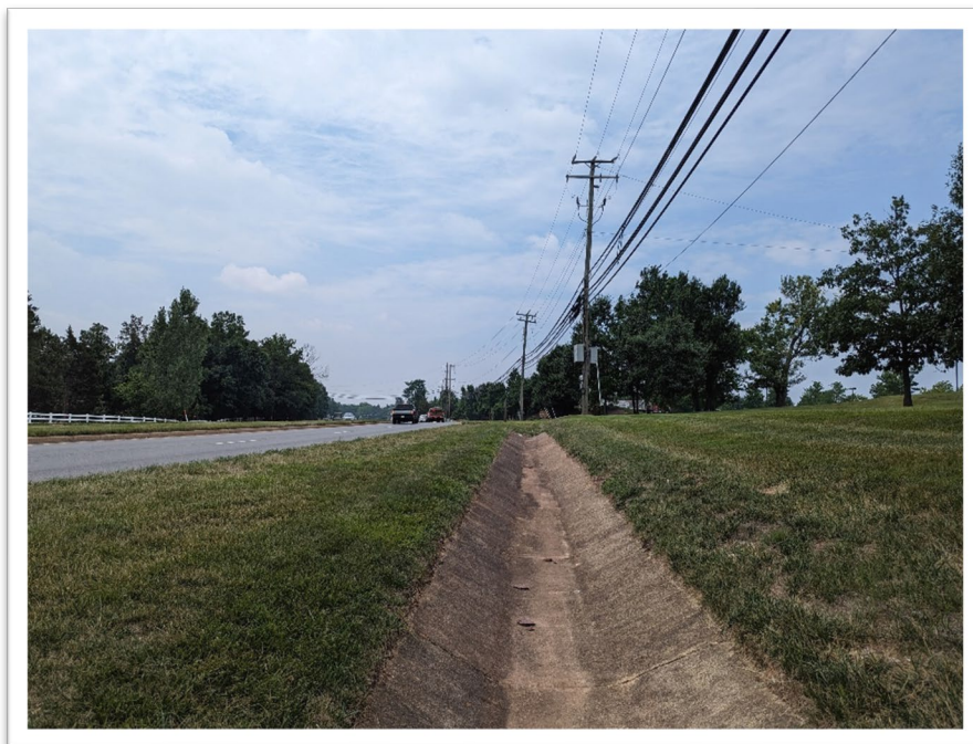
Field Photo 6: SB Cascades Pkwy looking south towards Oakbrook Court. Concrete ditch between Sta. 115+00 to 116+50.
