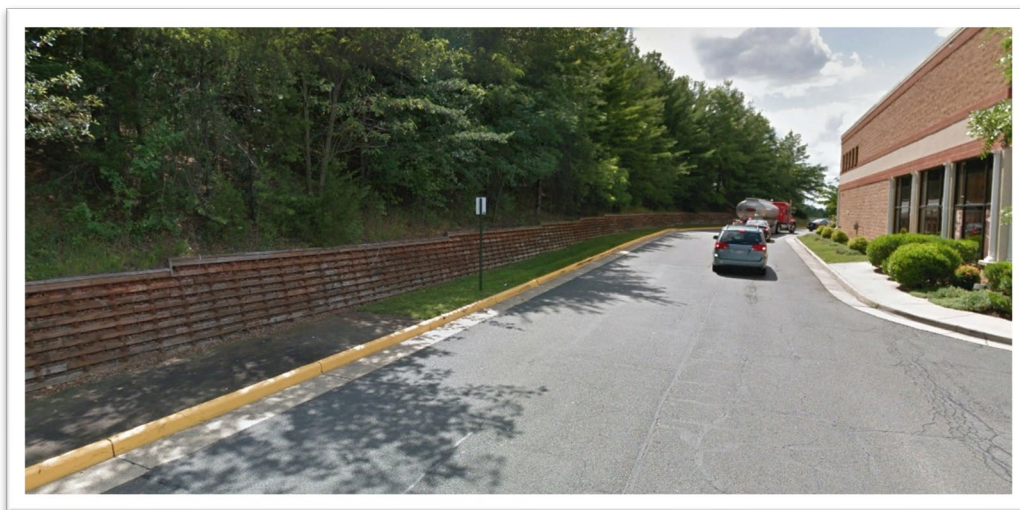
Field Photo 17: Price Cascades Plaza looking west towards Cascades Pkwy.
