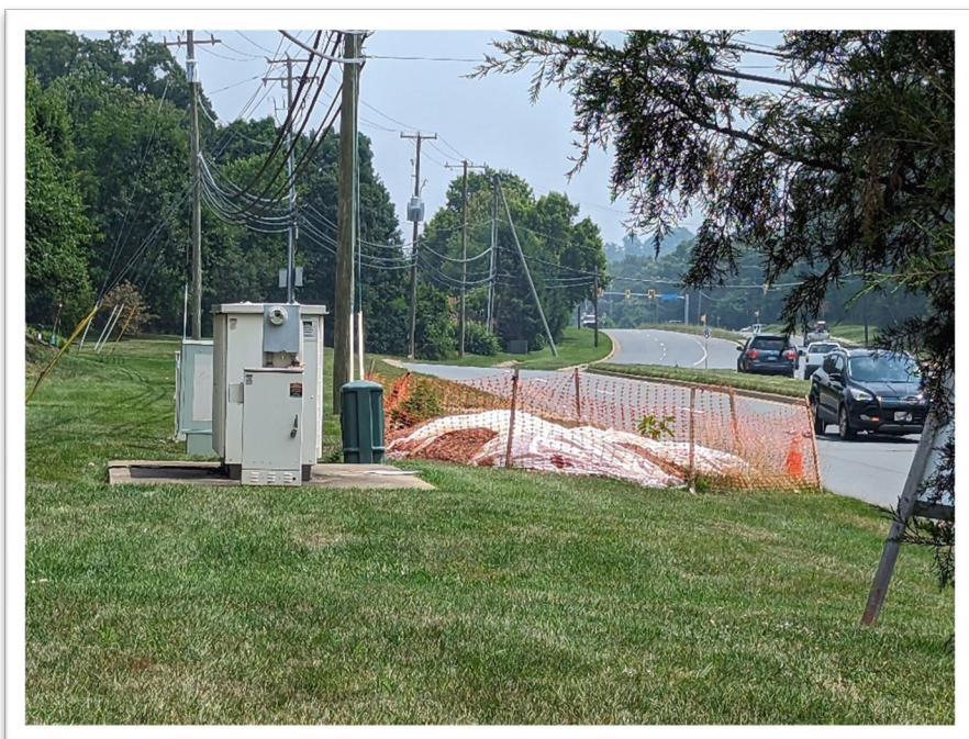
Field Photo 4: Cascades Parkway SB looking north at potential utility conflicts at Sta. 113+50.
