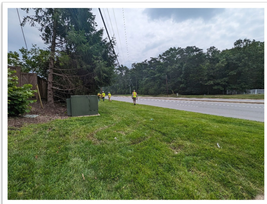
Field Photo 9: SB Cascades Pkwy looking north towards Victoria Station Drive at Sta. 121+50.00.
