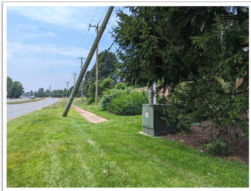
Field Photo 8: SB Cascades Pkwy looking south towards Oakbrook Ct. potential utility pole conflict at Sta. 121+00.00.
