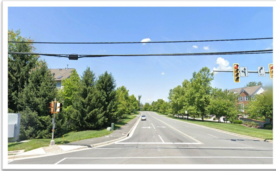
Field Photo 11: Cascades Pkwy looking west along Victoria Station Drive.
