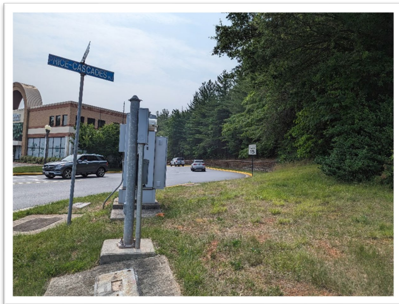
Field Photo 18: Traffic control cabinets at the southeast corner of Price Cascades Plaza.
