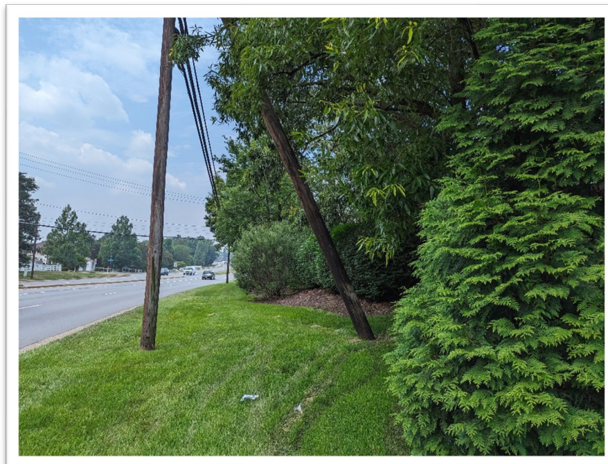
Field Photo 10: SB Cascades Pkwy looking south towards Oakbrook Court at Sta. 123+50.00.
