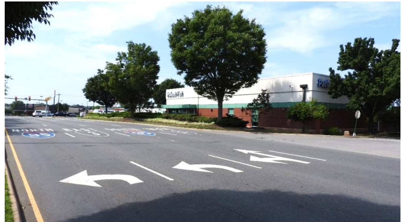
Figure 27: Carl D Silver Parkway (Looking south; Photo captured July 2023)
